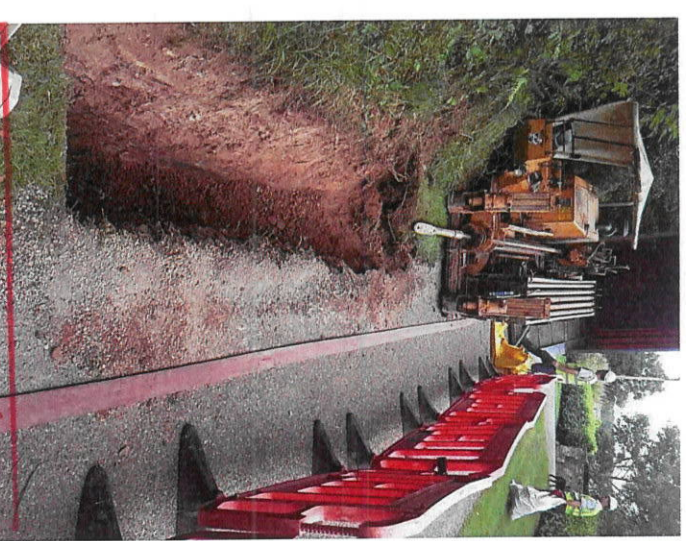
Image 2: Typical Directional Drilling Rig and Launch Pit
